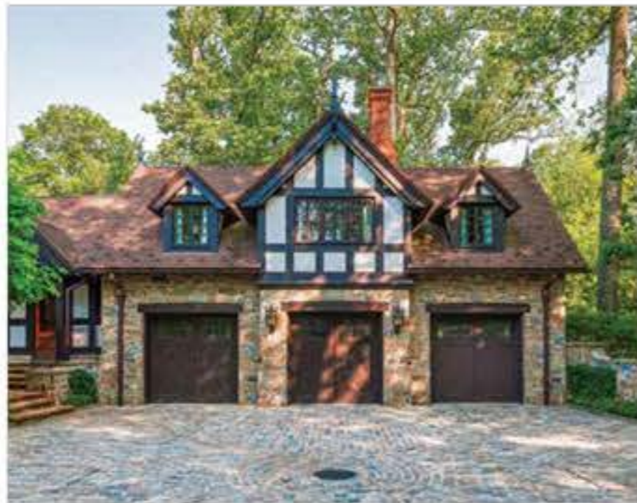
BOTTOM: The walkway between the garage and family room floods with natural light.
