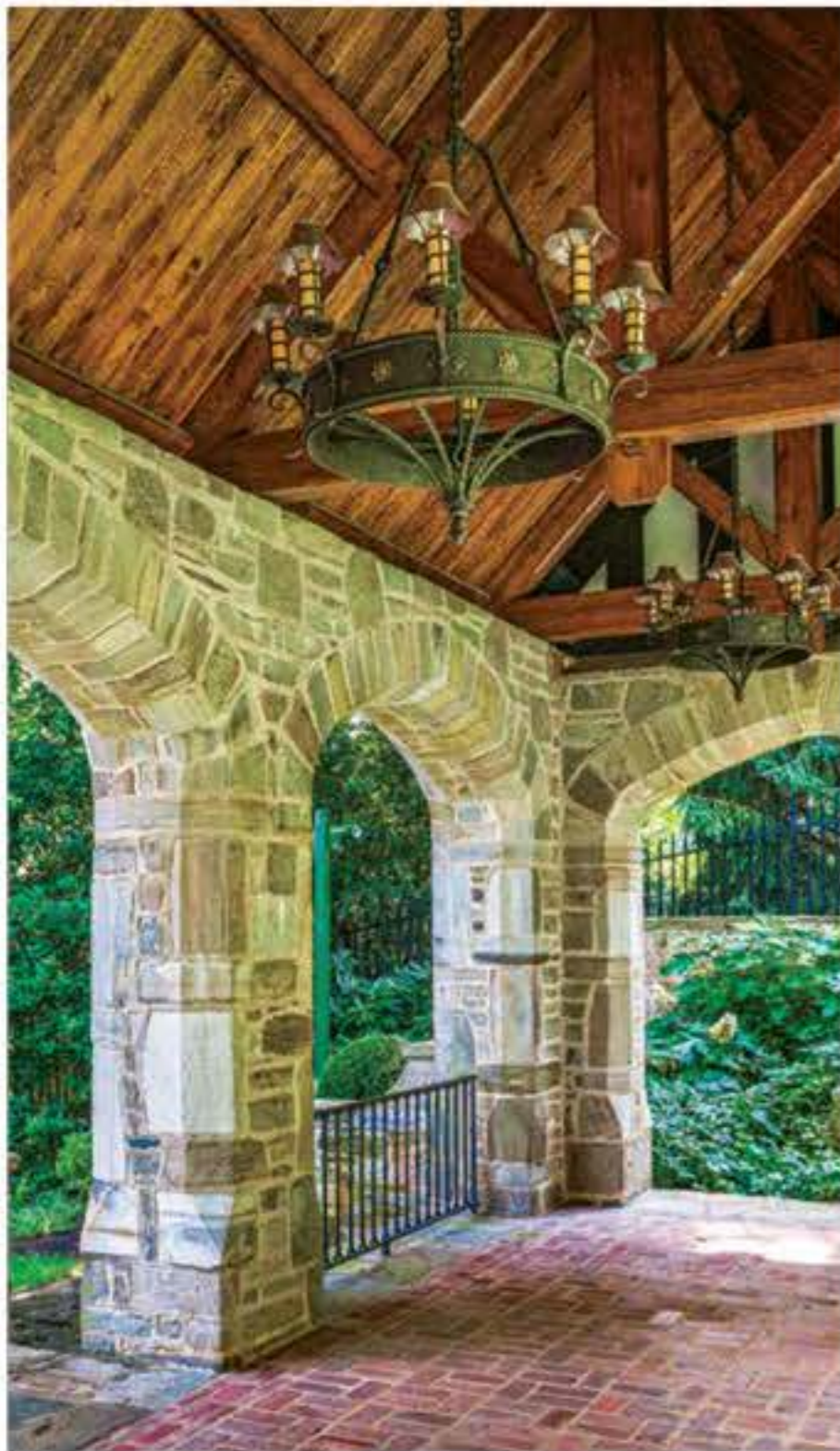
ABOVE: Sixty percent of the stone comes from the Rolling Rock Quarry. The remaining 40 percent was salvaged from an old carriage barn on the property as well as an old Main Line mansion.
