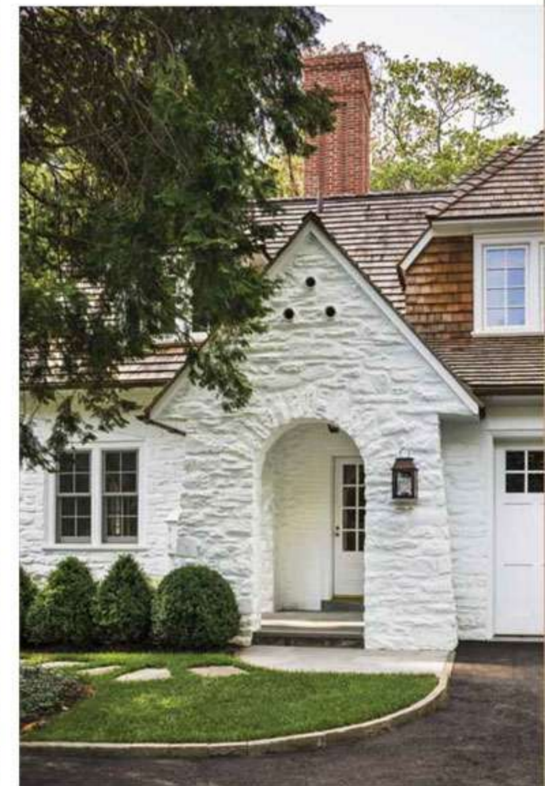
A secondary entrance, which leads from the new service court to the family living room, is defined by a stone arch and high-pitched roof.
