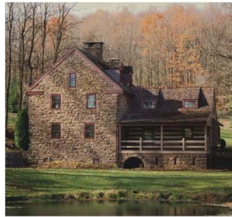
Above: A porch-fronted addition brings lofty family gathering space to a 1741 farmhouse. The new rosy fieldstone matches the original structure, and the new woodwork is salvaged barn boards. Photo: Peter Zimmerman Architects
